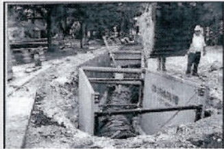
Crews work to replace the pipeline in Tampa.
